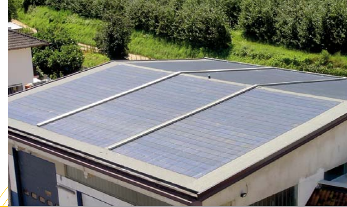
Commercial roof refurbishment with asbestos remediation, thermal insulation and double layer PHOENIX SOLAR waterproofing system with twenty-years warranty. 19 kWp General SOLAR PV building integrated photovoltaic system.
