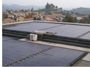
APPLICATION OF GENERAL SOLAR PV ON THE EXISTING ROOF, WITHOUT DRILLING THE ROOF
