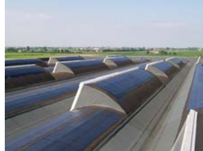
GENERAL SOLAR PV BUILDING INTEGRATED PHOTOVOLTAIC SYSTEM LAYED ON COUPEL AND SHED
