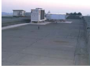
EXISTING ROOF WITH BITUMINOUS WATERPROOFING MINERAL MEMBRANE
