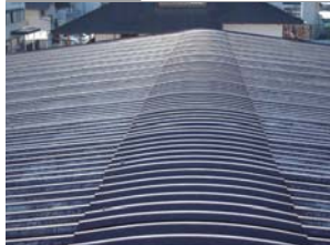
EXISTING ASBESTOS ROOF WITHOUT THERMAL INSULATION
