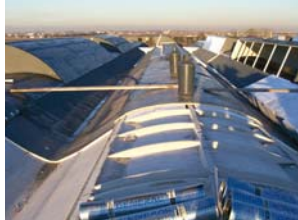
NEW BEAM, COUPEL AND SHED PREFABRICATED ROOF: WATERPROOFING WITH THERMAL INSULATION
