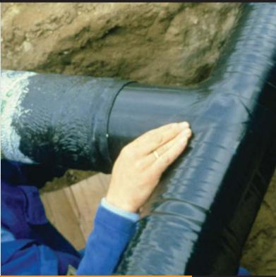
Anti-Corrosive Self-Adhesive Bitumen Tape
